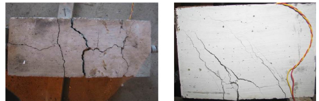
(a) View of beam base (b) View of beam side
